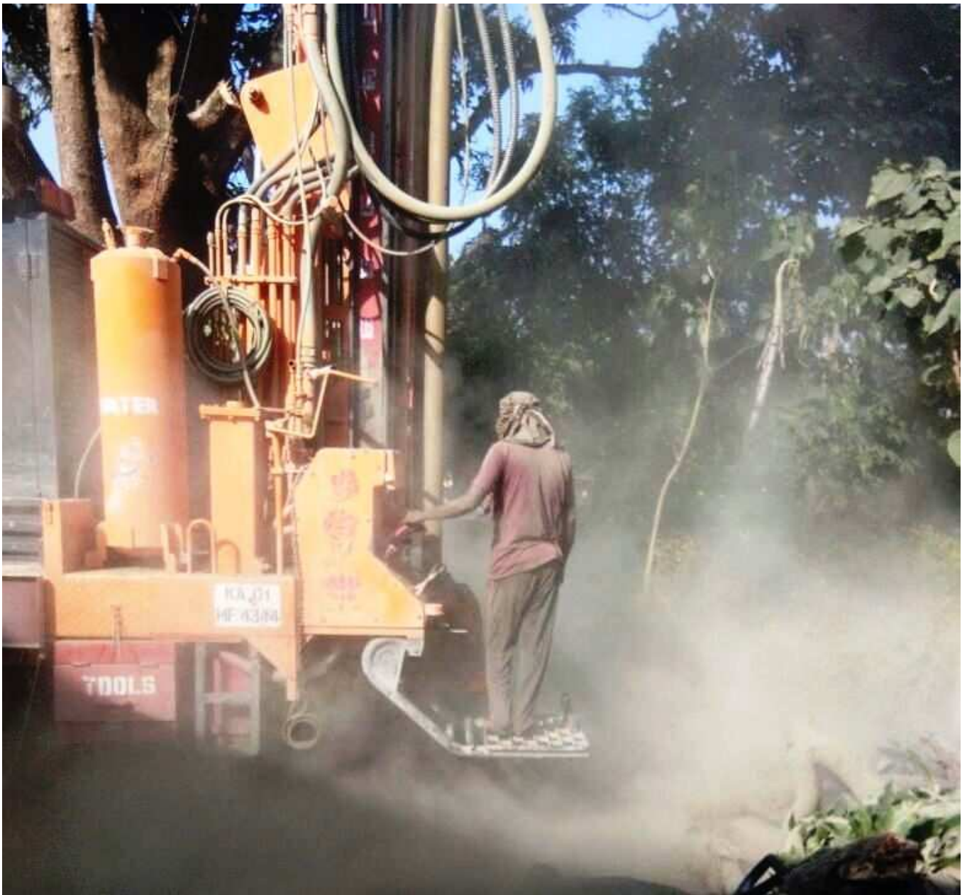
Drilling of deep bore well in progress (up)
